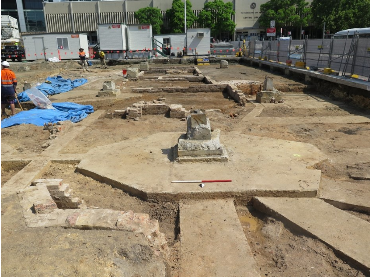
Figure 3.79: Detail of large concrete pads, piers and strip footing beams of the Post Office building in the northern end of the site in Areas A and B. View to the south, 1m scale. IMG_2930.
