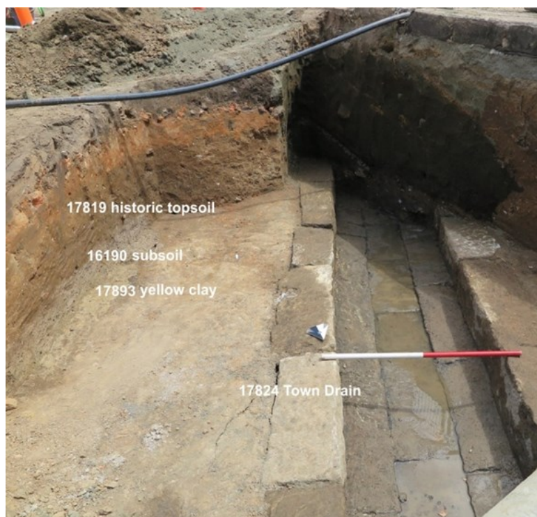
Figure 3.4: Natural soil profile emerging to the east of the edge of the cut for the drain. View to the south, scale 1m. IMG_5516.
