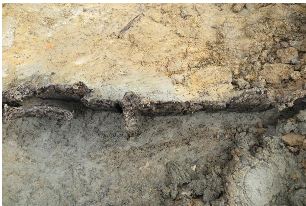
Figure 3.12: Detail of the timber barrier delineating the two deposits, showing an upright post perpendicular to the slabs. View to the west. IMG_5820.
