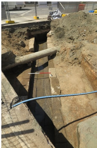
Figure 3.33: Southwestern end of sandstone Town Drain (left). View to the north. IMG_5755. Northeastern end of drain going under Macquarie Street (right). View to the north, 1m scale. IMG_5522.
