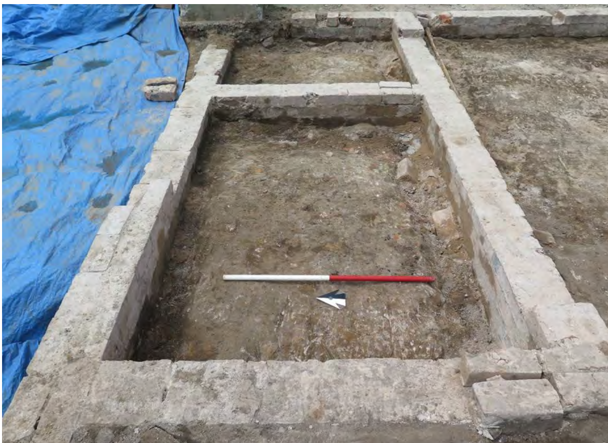
Figure 8.23: Breakfast room (Room 4a) in foreground and pantry (Room 4b) in the background. The demolition material has been removed down to the top of pre-construction fill 16124. View to the east. Scale 1m. IMG_2915.
