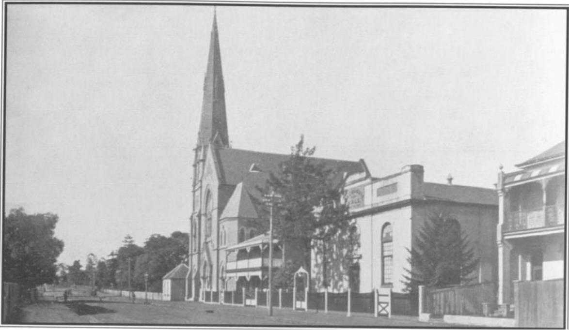
Figure 5.13: View to southeast, showing the buildings on Macquarie Street, west of Leigh Memorial Church, the parsonage, and Macquarie Hall. While none of the houses from Lot 30 or 32 are visible they do show the nearby streetscape to compare with Figure 2.23, Figure 2.26. McClymont 2003:20.
