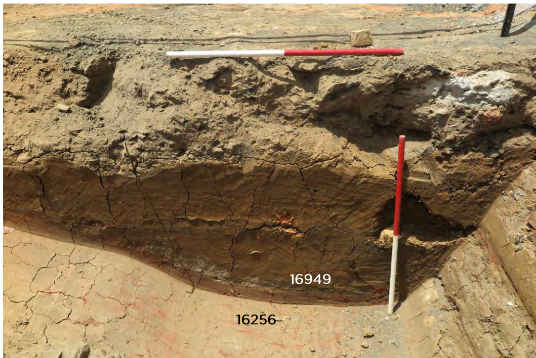
Figure 3.22: Section through the edge of the dam in the southwest corner of 3PS (TT14) exposed two layers of dense clay (16949 & 16256). Above the lower red and grey mottled zone (16256) was a gradual change to a yellow brown clay (16949). View to east, scale 1m. IMG_3704.
