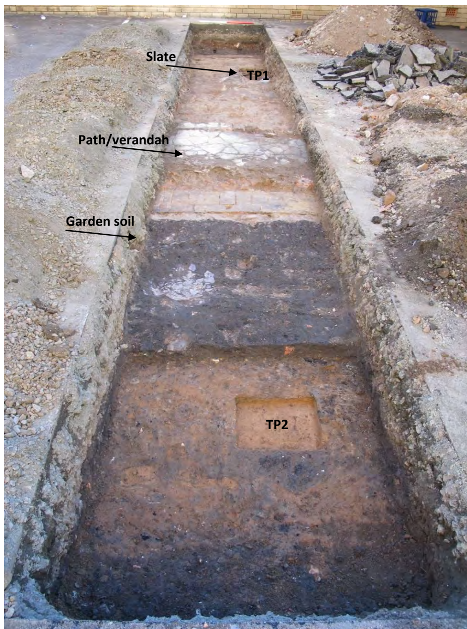
Figure 5.5: Trench A, view to the west with Test pit 2 in the foreground, and footings and verandah in the middleground. Compare with Figure 2.1. C&L 2013.
