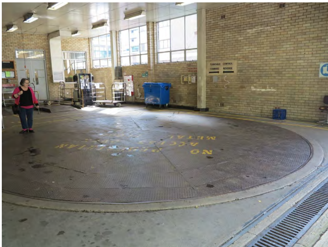
Figure 1.9: Truck turntable immediately inside the rear of the Post Office building. There is an excavated void approximately 400mm deep beneath the turntable for the machinery and clearance.
