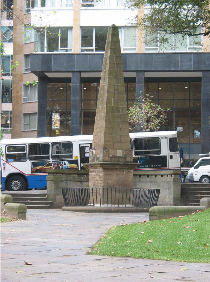
Figure 2.3: Obelisk looking east towards Loftus Street.
