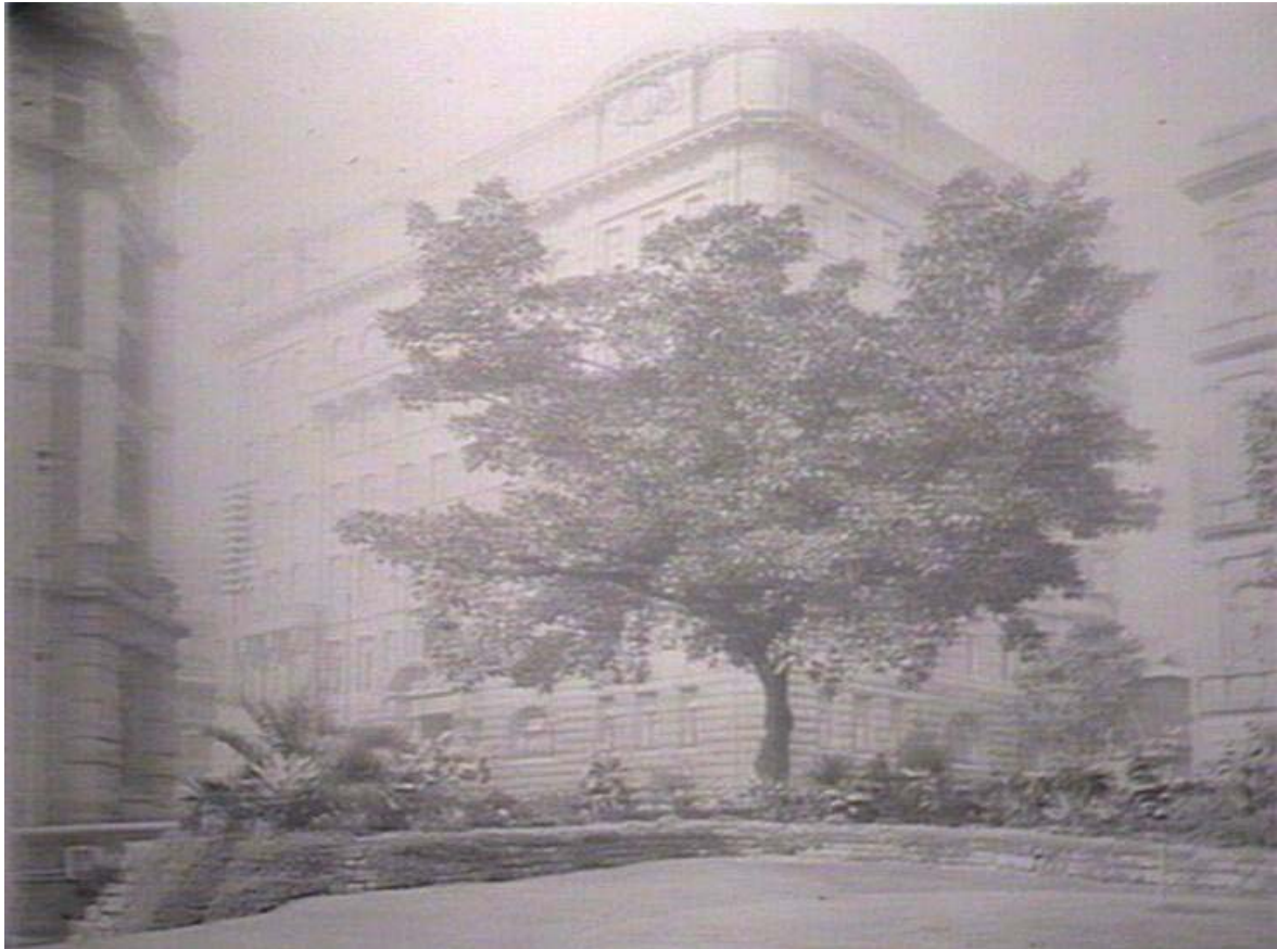
Figure 3.17: Raised flower beds at the corner of Bridge Street and Loftus Street May 1915, GPO 1-16214 (Mitchell Library).
