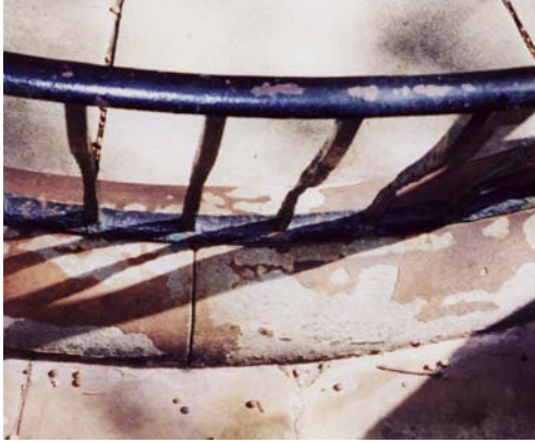
Figure 6.12: Dwarf wall of perimeter fence showing fretting from rising damp, April 2003.
