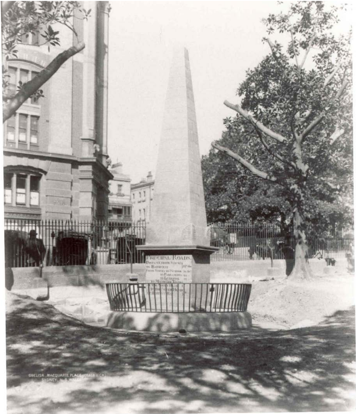
Figure 3.13: The back of the obelisk c.1895-1901. The area around the monument has been excavated to reduce ground level and the stone kerb is new (GPO 1-12583).
