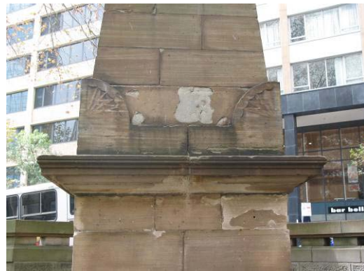
Figure 6.6: West cornice and acroterion course, April 2003.
