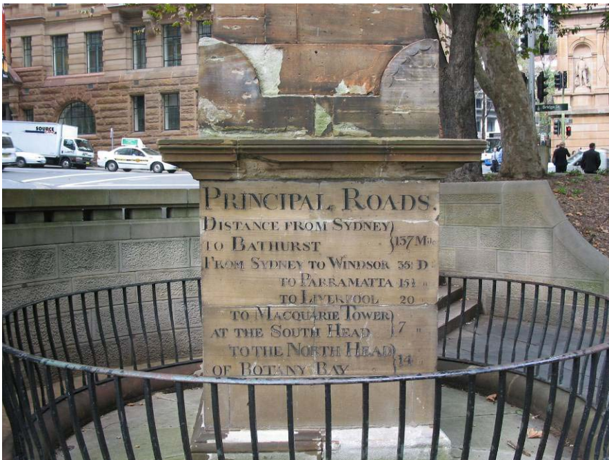
Figure 2.5: Northern face with one of two panels of inscription. The pedestal base is exfoliating. Only one of the two visible acroteria has the carved fan decoration and the other is blank.
