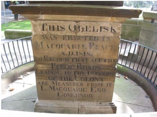
Figure 6.7: Southern pedestal showing fretting and variation of colour in courses, April 2003.
